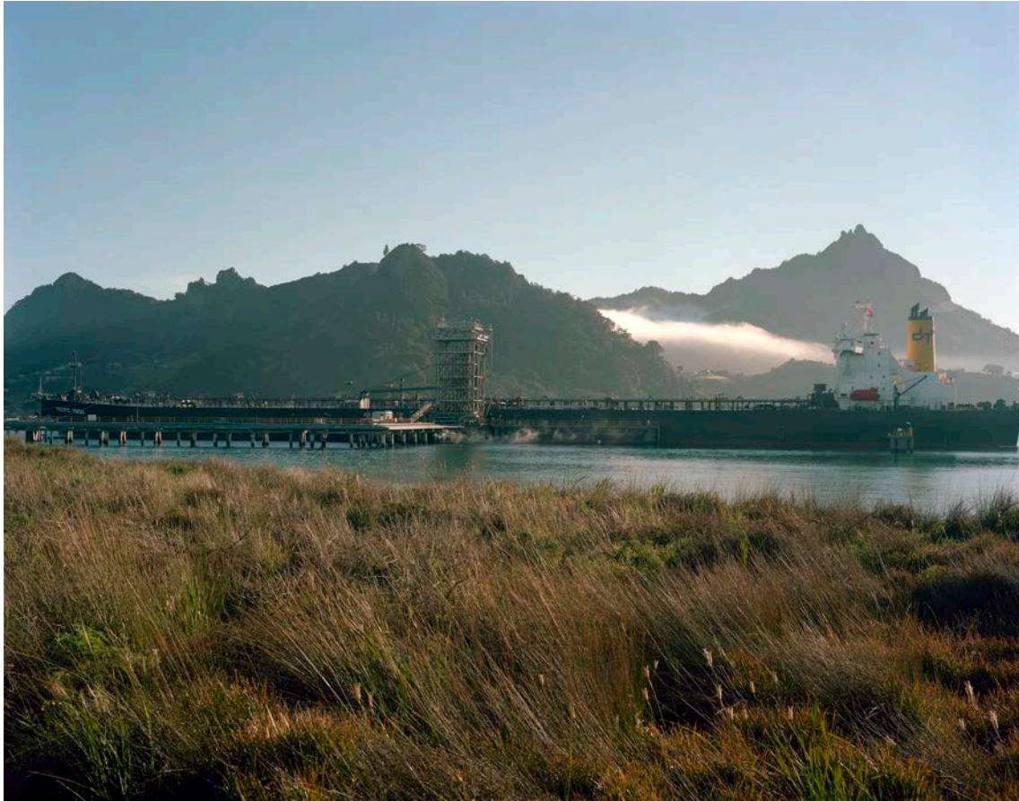
Oil Tanker, Marsden Point, Whangarei, 28th August 2011
