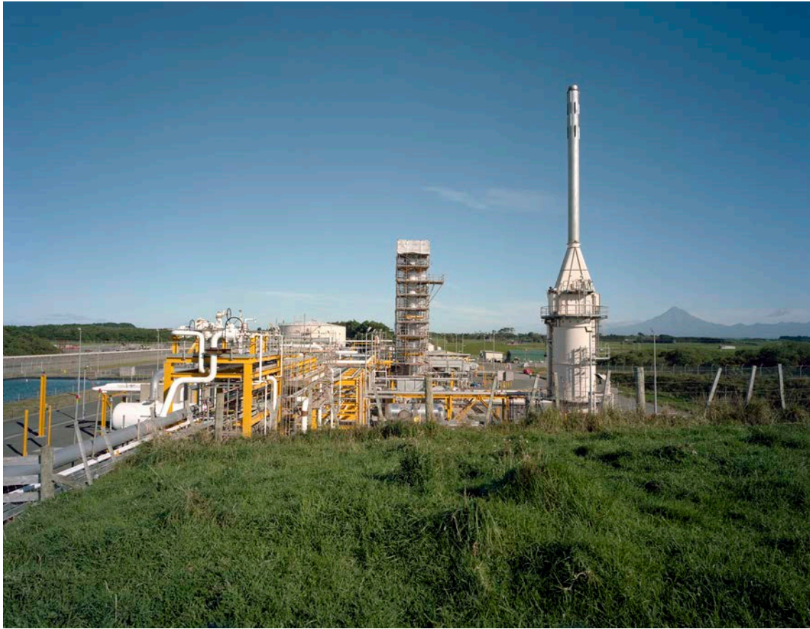
Pohokura Production Station, Motunui, 18th April 2012
