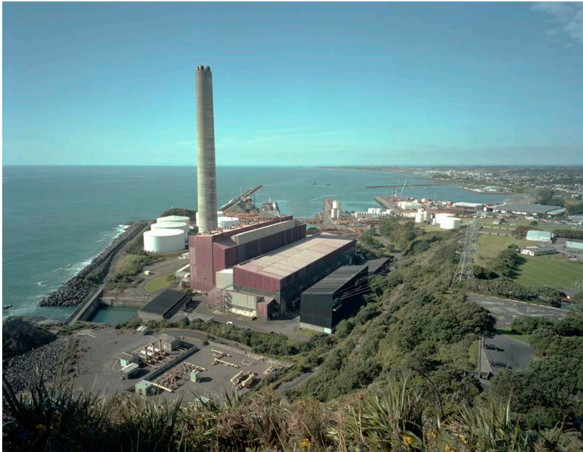
New Plymouth Power Station, Port Taranaki, New Plymouth, 17th April 2012
