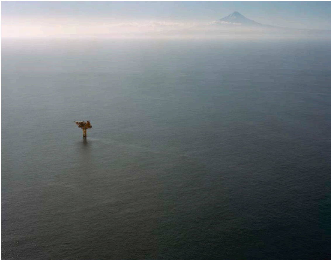
Kupe Natural Gas Field (unmanned Wellhead Platform), Tasman Sea, 20th July 2012
